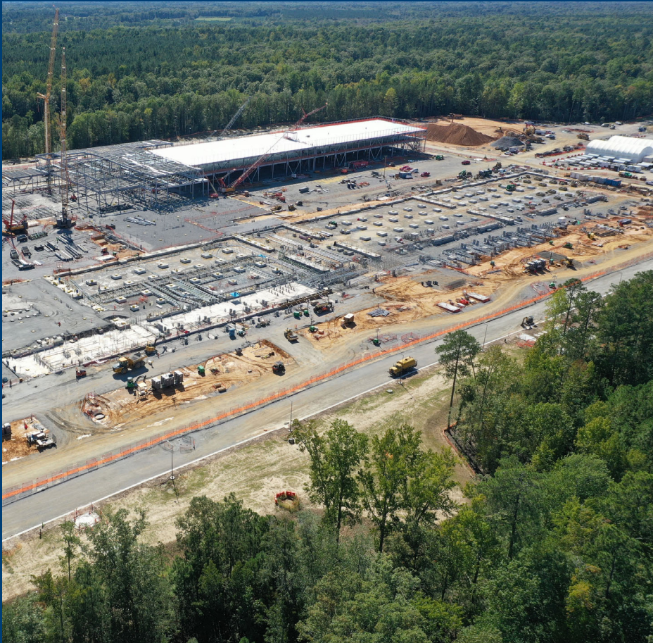
FACEBOOK DATA CENTER – CENTURY CONCRETE
